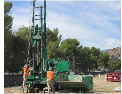
Drilling rig used to install air sparging system in early 2015
