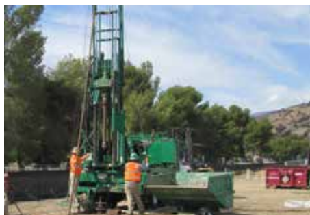
Drilling rig used to install air sparging systems
